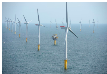
(b) Wind power facility
