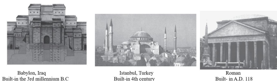
Figure 4. Historical structures constructed using lightweight aggregate [21].
