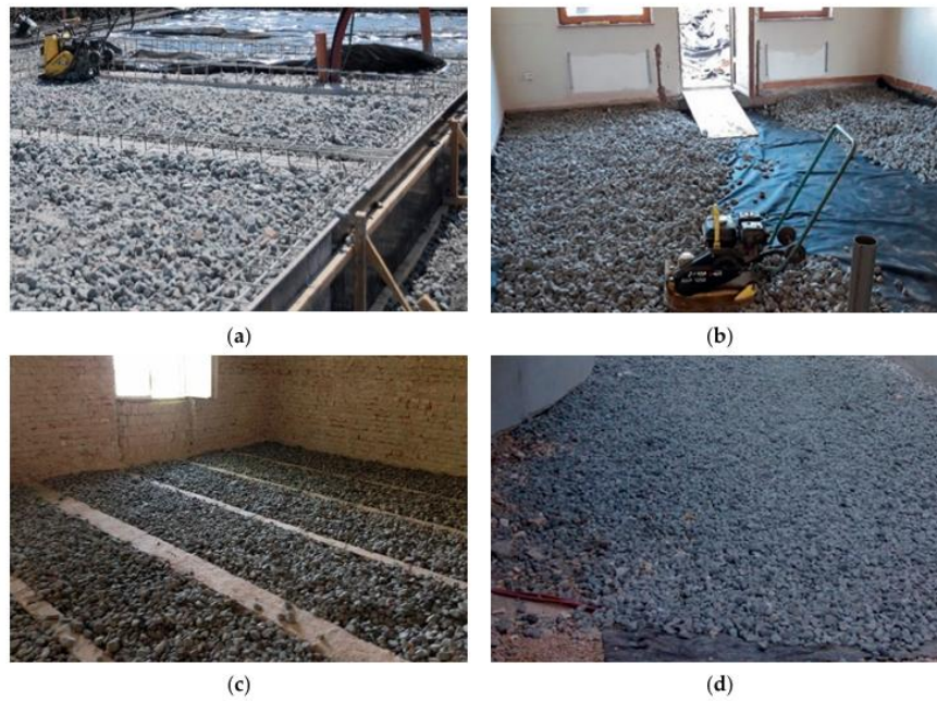
Figure 7. Foam glass aggregate applications: a) insulation of ground-contact slabs, (b) slab insulation during building refurbishment, (c) insulation of intermediate slabs in refurbishments, and (d) base and insulation layer for heated underground garage ramps [30].
