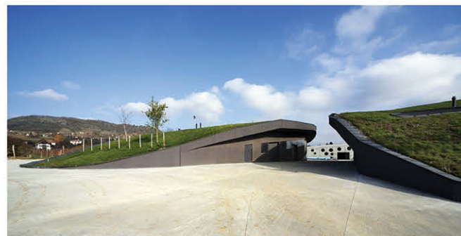
FIG. 8. BACK VIEW OF THE ST.ILONA WINERY AND KREINBACHER CHAMPAGNE WINERY
