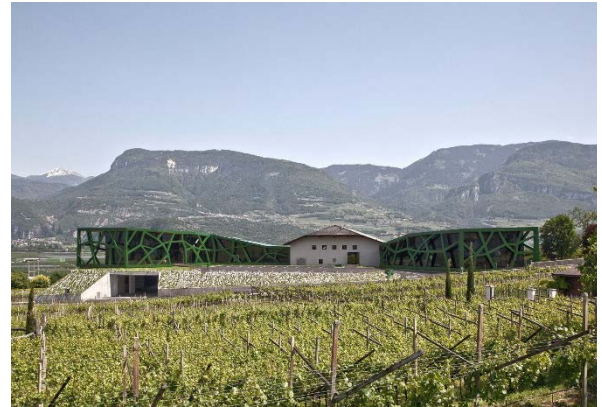
Fig. 4.52. General view of the Tramin Winery (4.300 m 2 | 2010 | IT)
