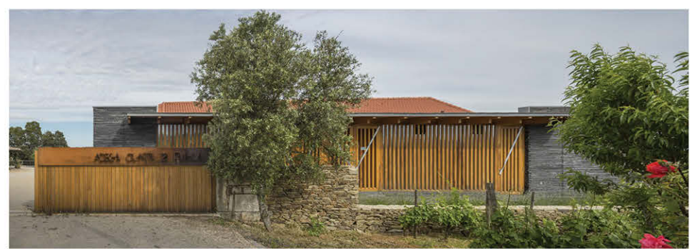
FIG. 7. SIDE VIEW OF THE EXTENTION, REFLECTING THE USED MATERIAL
