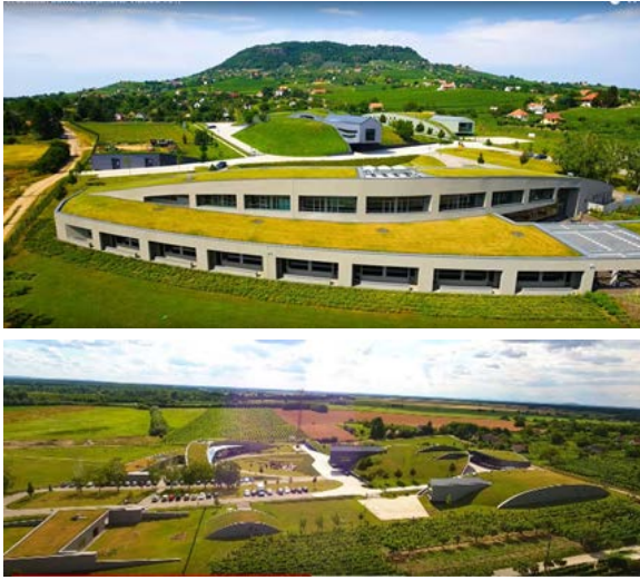
Fig. 4.11, 4.12. Bird's eye views of the Kreinbacher-St. Ilona Winery complex (5.947 m 2 | 2012-2104 |
