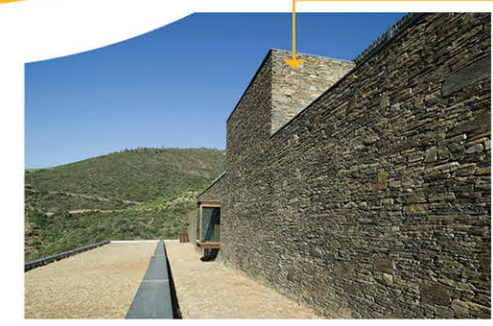
FIG. 6. CLOSE VIEW OF THE WINERY, WHICH REFLECTS THE USED MATERIAL, PANORAMIC WINDOW AND THE VIEW FROM ITS ROOF WHICH IS OFFERED TO VISITORS
