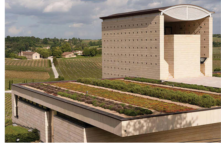
FIG. 6. CLOSE UP VIEW OF THE WINERY, REFLECTING THE TEXTURE OF THE MATERIAL, GREEN ROOF AND THE VIEW TOWARDS THE OLD CHATEAU
