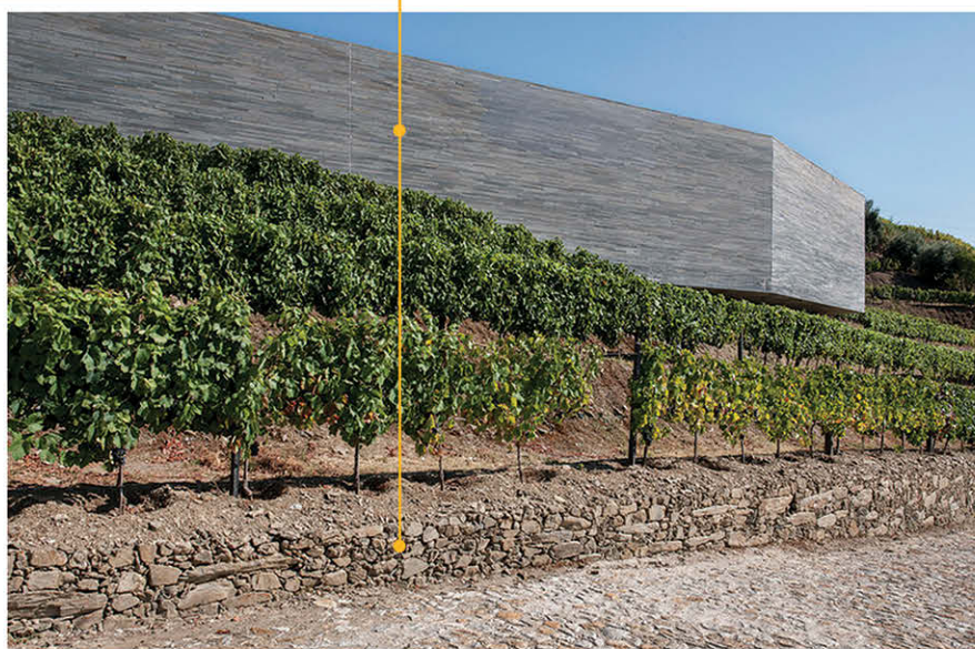
FIG. 8. DETAIL VIEW OF THE BARREL WAREHOUSE (CELLAR) AND THE STONY TERRACE ON WHICH THE VINES GROW
