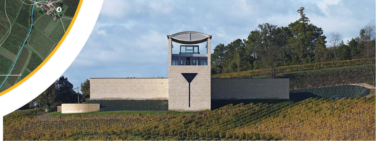
FIG. 5. FRONTAL VIEW OF THE NEW WINERY, REFLECTING ITS SHAPE AND USED MATERIALS
