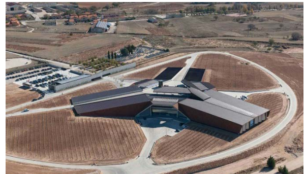
Fig. 4.54. Bird's eye view of the Faustino Winery (12.500 m 2 | 2010 | ES)
