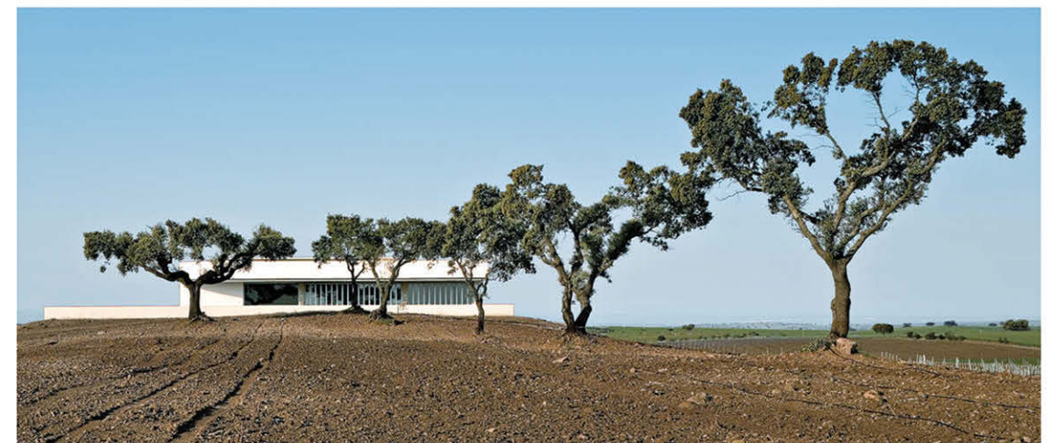
FIG. 5. BACK VIEW OF THE WINERY AND ITS NATURAL AND CULTURAL CONTEXT
